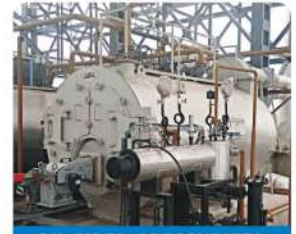
OIL FIRED PRESSURIZED HOT WATER GENERATOR
